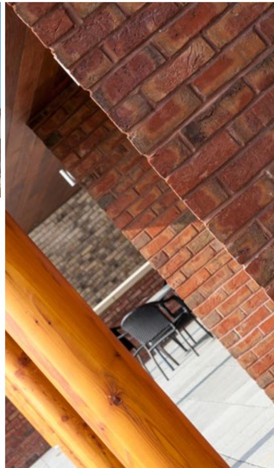
A noticeable feature of the property's exterior is its creative use of Wienerberger's Loxley Red Multi bricks, which envelop the insulated concrete formwork system employed as the mainstay of the wall's load bearing capacity and thermal efficiency.
